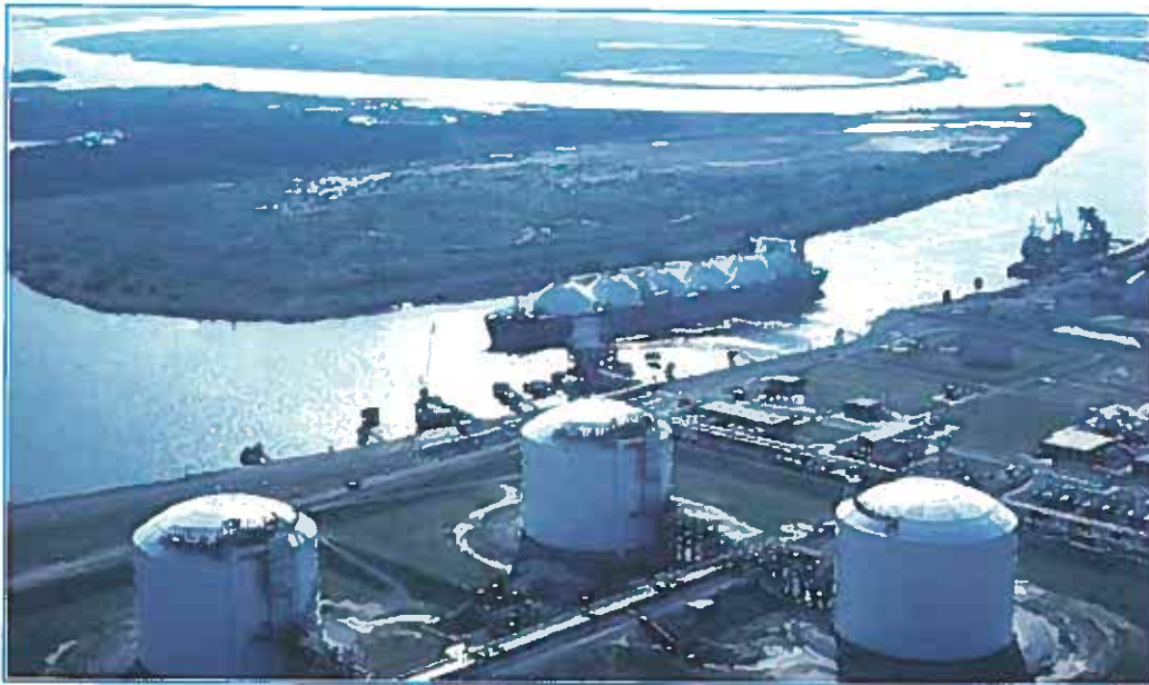
Lake Charles Import Terminal, Louisiana
